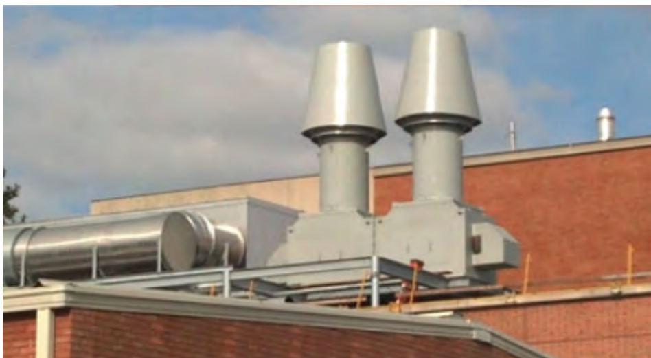
The PennBarry Hy Plume nozzles shown above are like those that will be installed on the laboratory buildings at the new KSU Girls campus.
