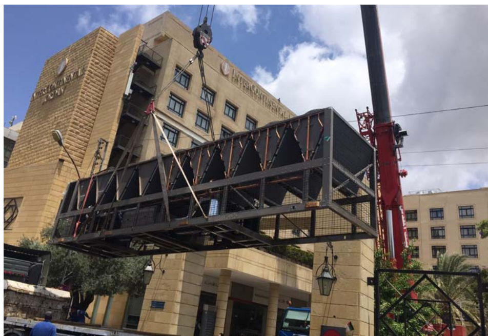
Workers install the new chiller on the roof of the Intercontinental Hotel in Amman, Jordan.
