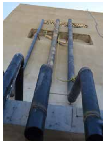
Workers install the massive piping layout for the steam boiler system being installed at the new Serum & Solutions plant being constructed in Saaraain, Baalbeck, Lebanon.
