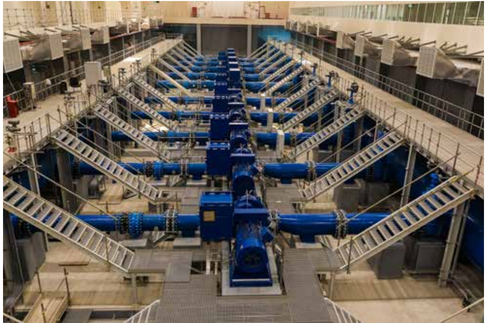
BLE fire curtains are designed to deploy along the row of control room windows (upper right in photo) overlooking the massive pump station. The curtains will protect occupants in the control room in the event of a fire in the pump station.
