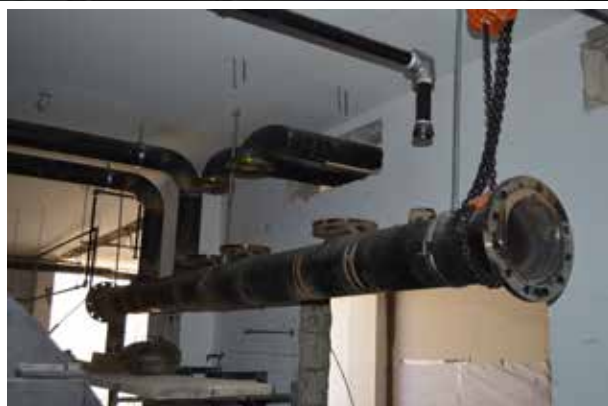
Workers install the massive piping layout for the steam boiler system being installed at the new Serum & Solutions plant being constructed in Saaraain, Baalbeck, Lebanon.
