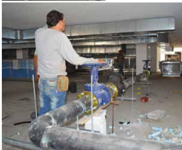
Workers install the massive piping layout for the steam boiler system being installed at the new Serum & Solutions plant being constructed in Saaraain, Baalbeck, Lebanon.
